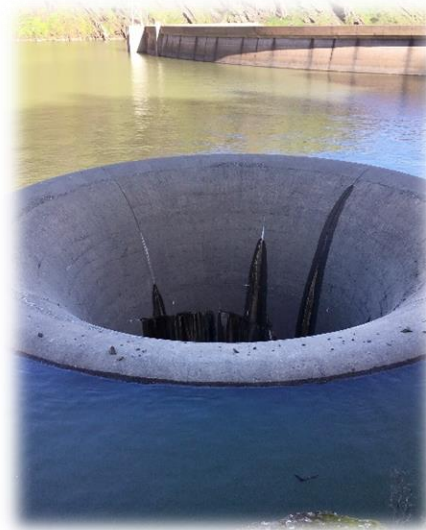
Secondary outlet – riser / spillway
