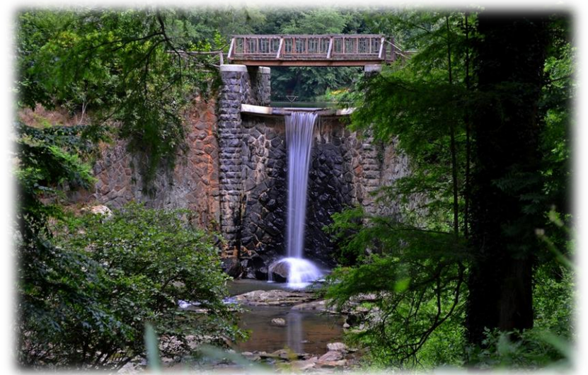
Secondary outlet – riser / spillway
