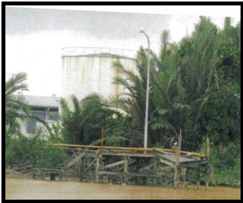
Power Plant Jetty
