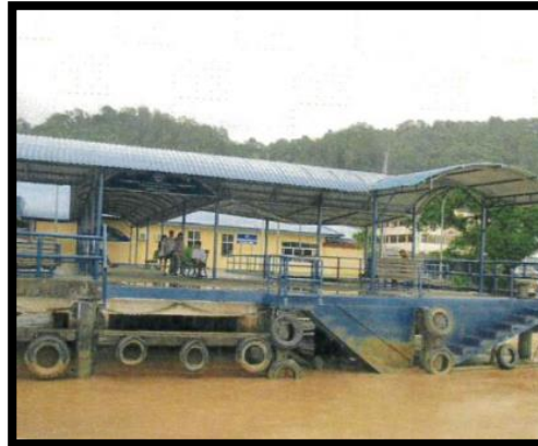
Jetty for ferry landing at Custom Wharf
