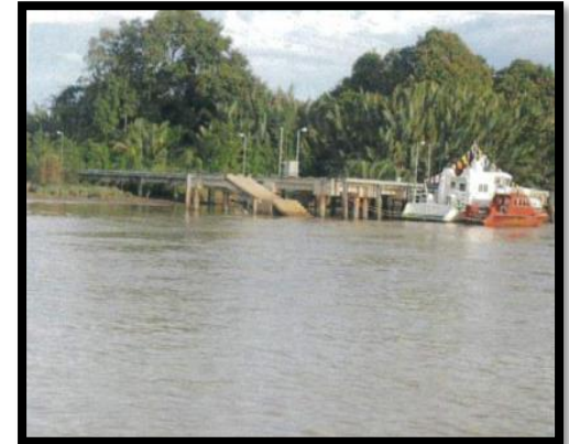
Jetty for ferry landing at Custom Wharf
