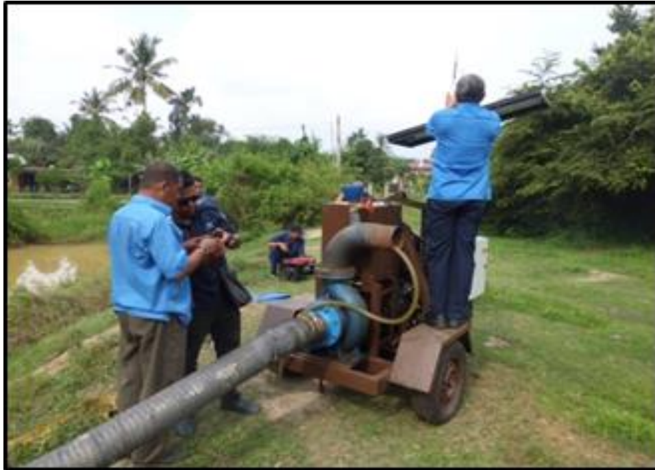
Gambar 8 : Pemasangan Remote Control Mobile Pump (RCMP) di tapak.
