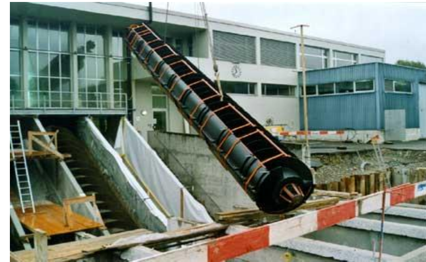
Steel trough liner (assembled to the screw body)
