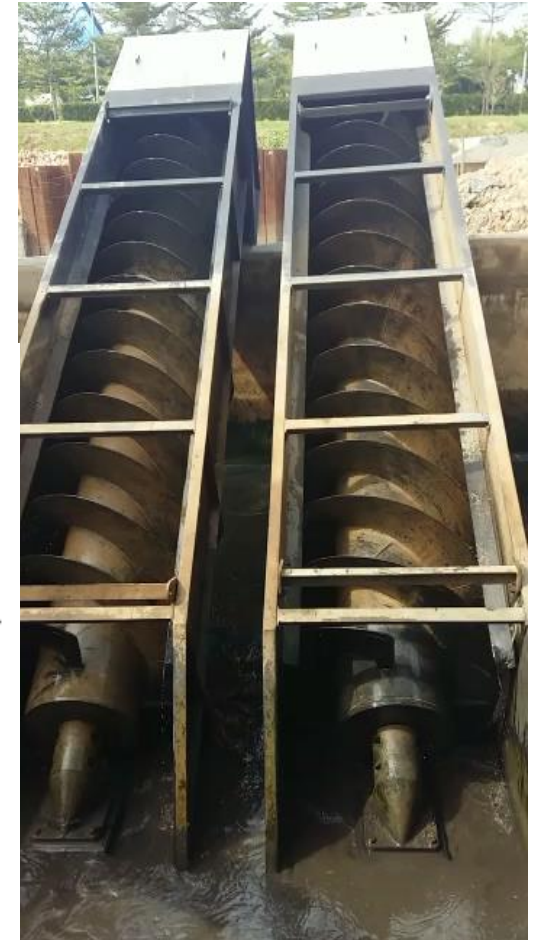
*video of screw pump running in dry condition.
